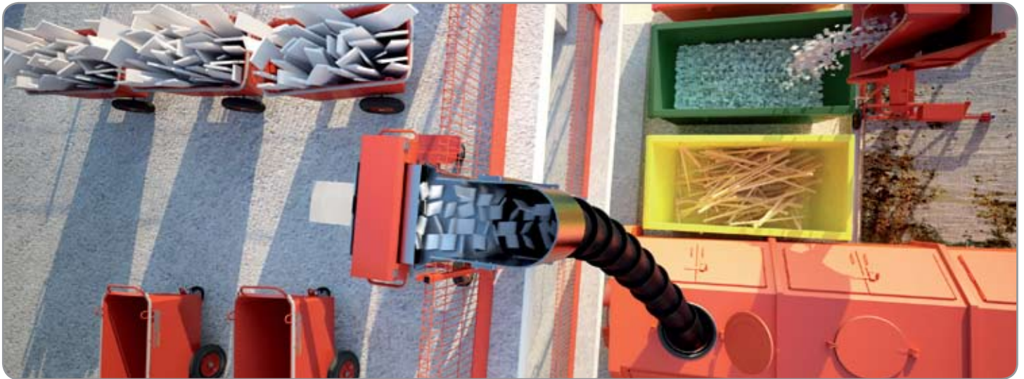
The chipper gives the option of using a waste chute within the building therefore reducing on site handling
